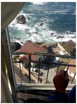
The first steps will be to remove these windows and then string a wire from the tower down to the Fog Signal Building (pictured). Once the wire and hoist are secured then they will be ready to bring down the secured lens panels. This Steve and his crew are doing this Jim Dunlap (The Lampist) and his crew with be carefully taking the panels apart from one another and packaging them for transport.
