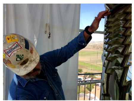
Even with all of his experience, Steve stood amazed at the 24 bulls-eye lens of the Pigeon Point Fresnel Lens – "Much more then most". Here Steve sizes up the individual lens panels, which will be removed, packaged and then hoisted directly down to the Fog Signal Building.
